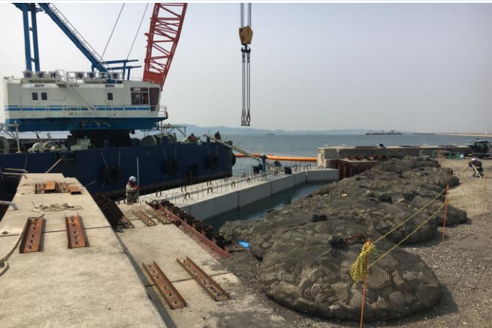
Seawall repairing & raising
